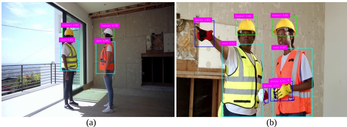
Figure 7. Examples of PPE detection results using the YOLOv11s architecture: (a) safety helmet and vest detection; (b) gloves, safety helmet and vest detection
